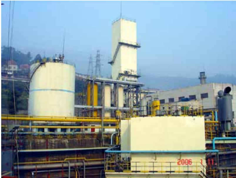
Air Separation Plant in Panzhihua
